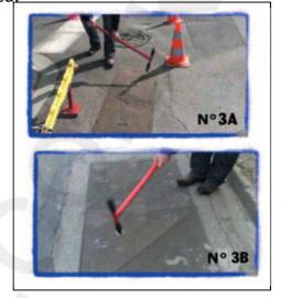
**4)** Commence by lifting out an end plate. To do this, position machine in front of or as near to the centre of gravity of the plate concerned, lift and roll.
